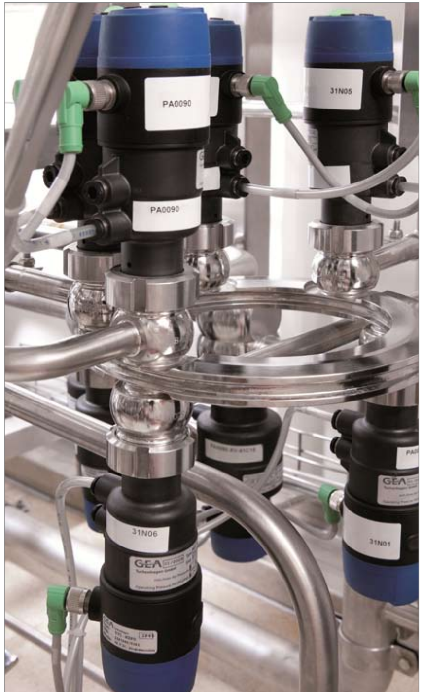
The multiport ring distribution systems of the VESTA® series are free from any dead space and are characterized by their compact design.
